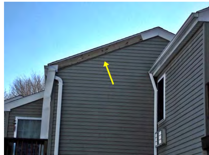
A storm-damaged fascia board (scheduled to be repaired).
