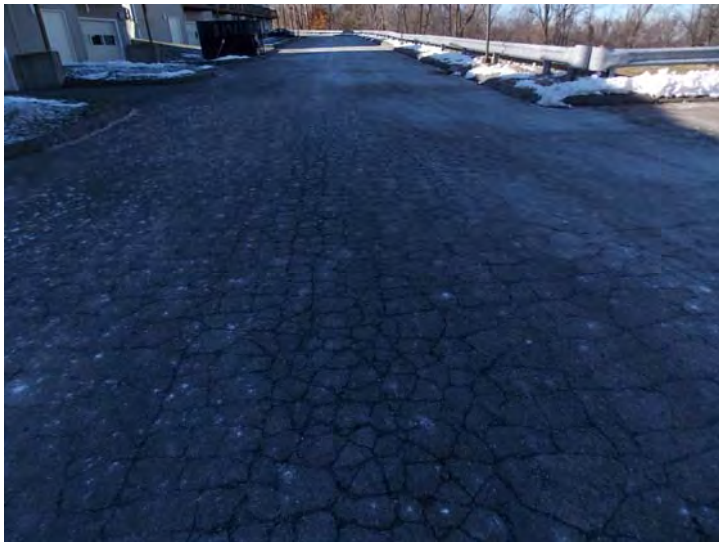
Asphalt paving has a series of cracks.
