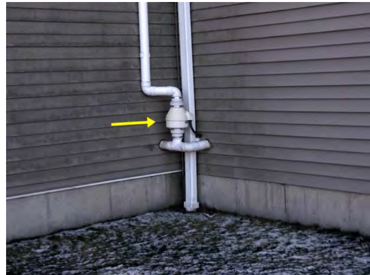
One of the radon gas abatement systems.
