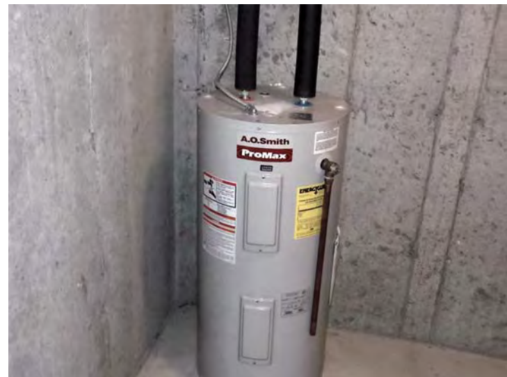
Each apartment has its own electric-heated DHW tank, which is located in basement.
